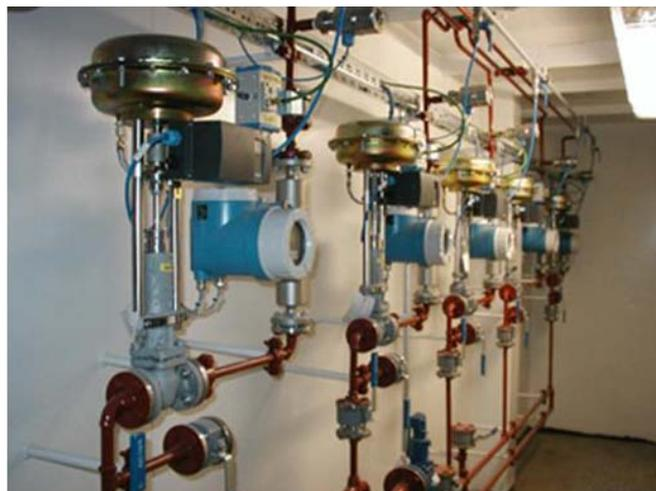
**Figure 4.28:** Measuring and dosing station with pneumatic valves
