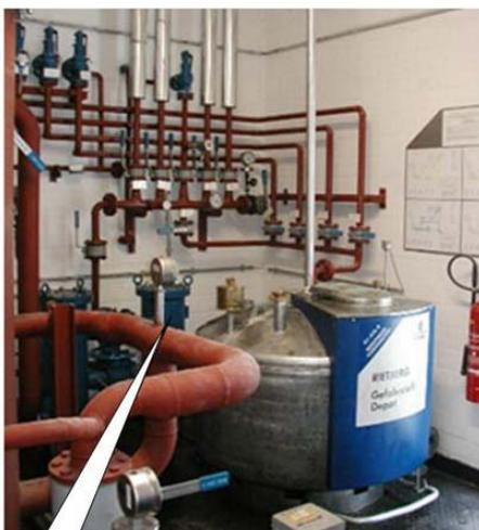
**Figure 4.27:** Pumping station number 2 with a filter and a waste container for cleaning the filter
